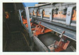
**Figure 4.** Technicians installed three impact cradles in the loading zones on each conveyor to create a flat edge for improved containment.
